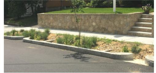
Curbed inlets allow water to enter the constructed bio-retention systems (photo courtesy of Horsley Witten Group).
