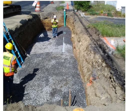
Tree trench underlain by gravel to enhance subsurface storage and increase rate of infiltration (photo courtesy of Horsley Witten Group)
